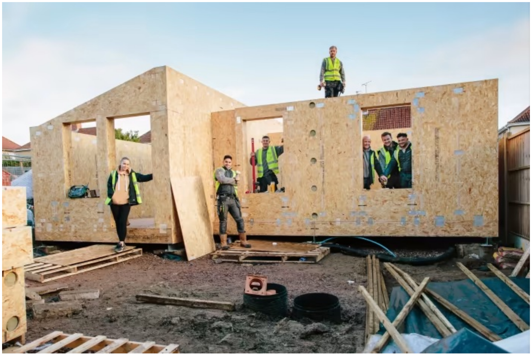
One of WeCanMake's units under construction © Ibolya Feher/WeCanMake
